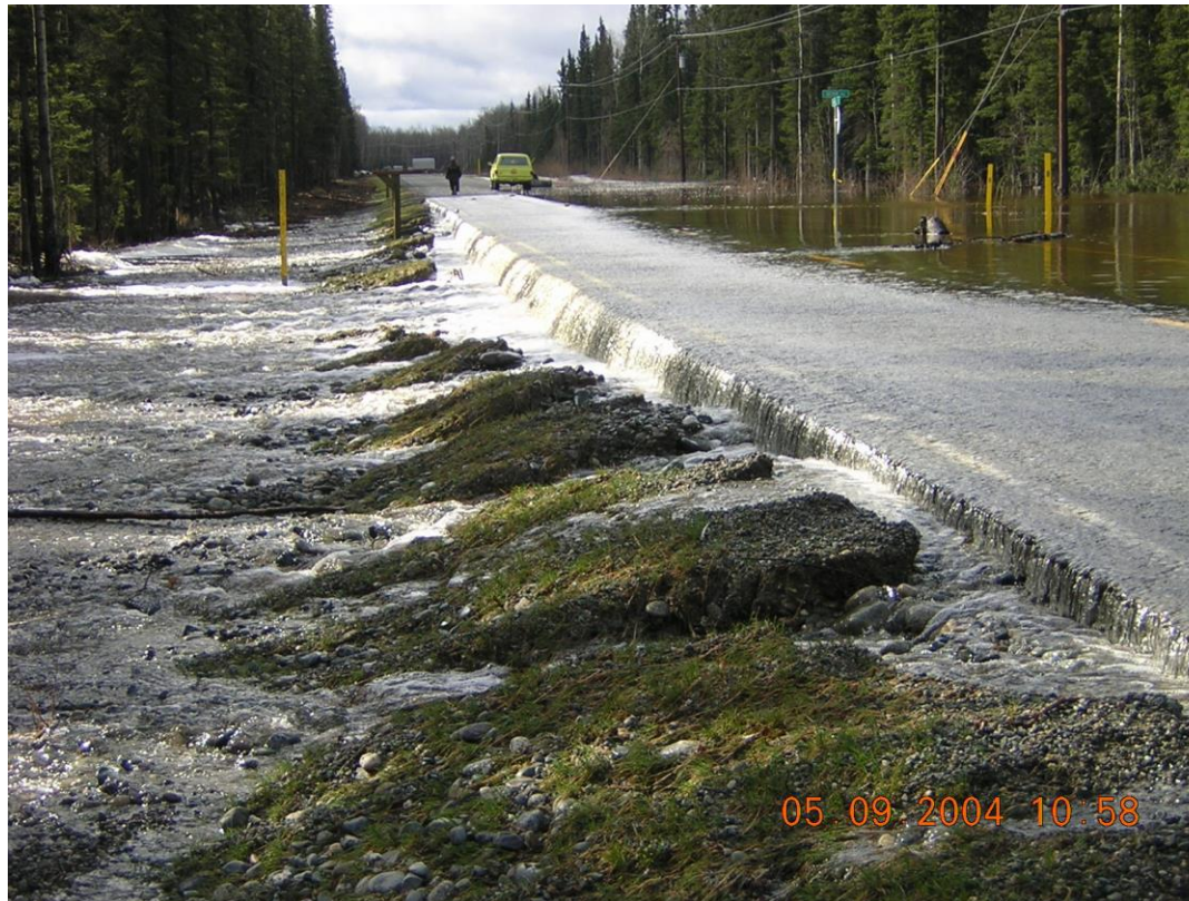
Undercutting at Berm Road (Delta)
